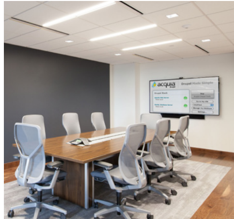
Via 5 recessed in a grid ceiling
